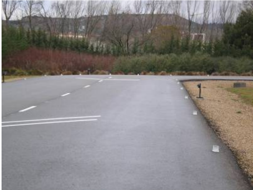
Image: Solar beacons on the edge of track in the non-testing zone.
